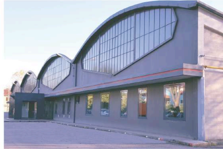
FABRICATION PLANT 2 NPD Noventa Padovana - Padova
