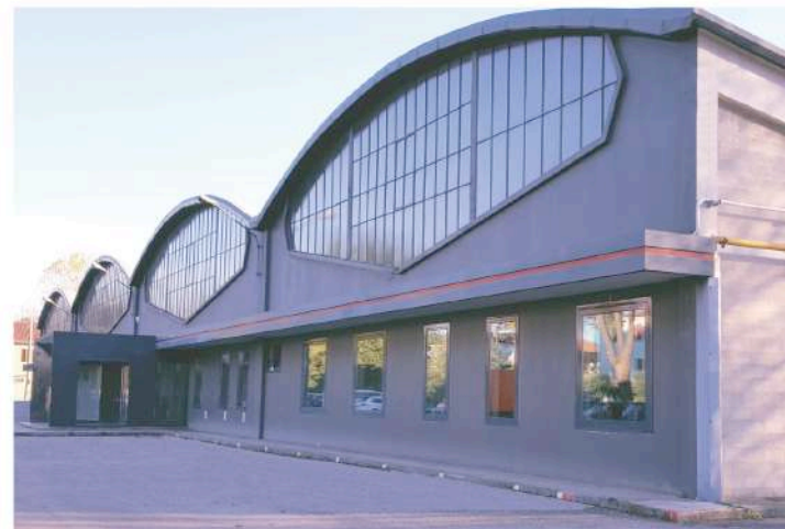
FABRICATION PLANT 2 NPD Noventa Padovana - Padova
